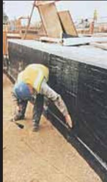
to provide an even surface. Concrete and render should be completely cured, dry and dust free. All areas must be primed with Alderprufe SA Primer at a rate of approximately 4-6m<sup>2</sup> per litre prior to the application of Alderprufe MR50 and allowed to dry. Only prime sufficient
